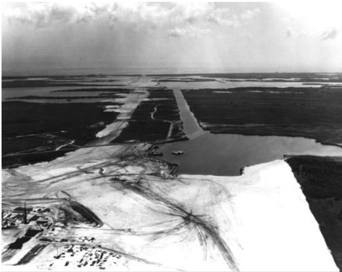
The barge canal and turning basin, with assembly building site in lower left, August 1963.
